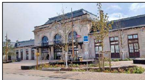
Gare multimodale et parking
